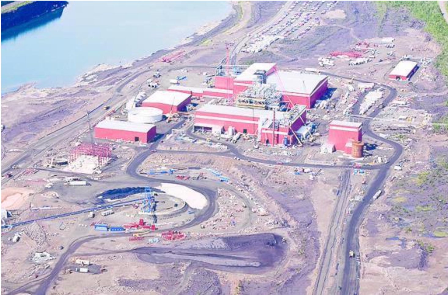
Aerial view of the 500kt/year ITmk3 plant in Minnesota operated by Steel Dynamics Inc. The plant was mothballed in 2015-2016. Image used with permission courtesy of Aaron Brown, www.minnesotabrown.com
